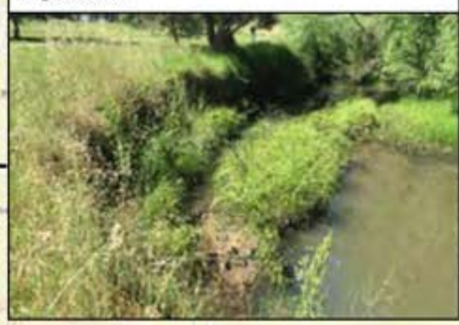
Bank Slumping and lack of stabilising bank vegetation.
