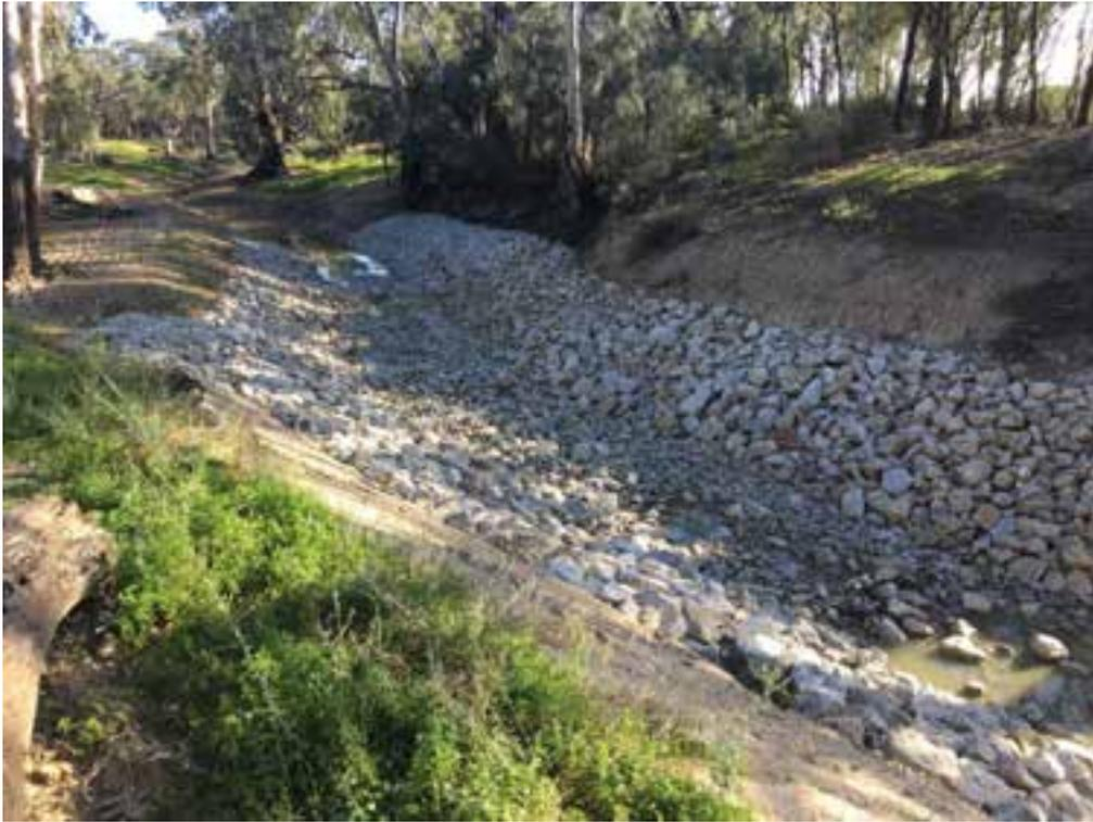
**Figure 6-5** An example rock chute, aimed at providing a stable bed gradient from one bed elevation to a lower bed elevation.
