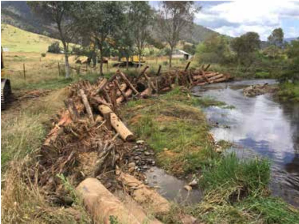
**Figure 6-4** An example of a timber revetment site, aimed at managing bank erosion. The application of this technique is strongly dependent upon the availability and arrangement of suitable timber.
