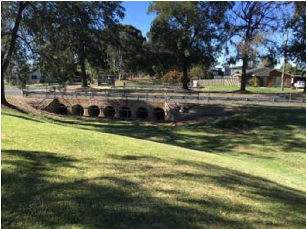
Figure 2-8 Constructed Floodway on Jack in the Box Creek.
